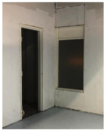
*Window 2:* Existing heritage window in poor condition. Currently covered by ATM services on the outside. View shown from inside existing building.
